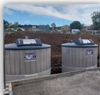
Conteneur semi enterré
